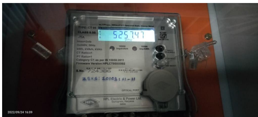
Figure 2: Energy meter
